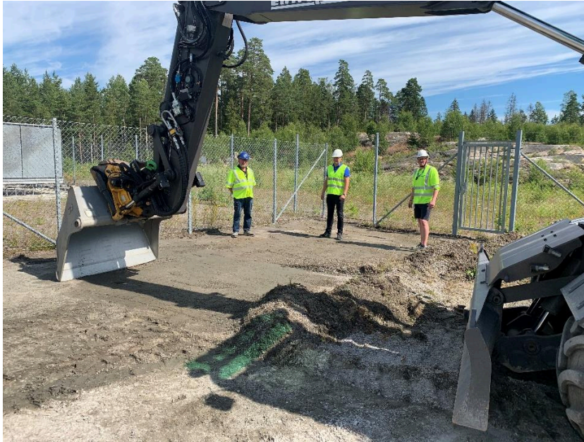
Start of civil work August 2020
