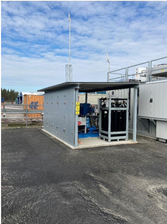
The compressor got a roof and a protection wall, June 2021
