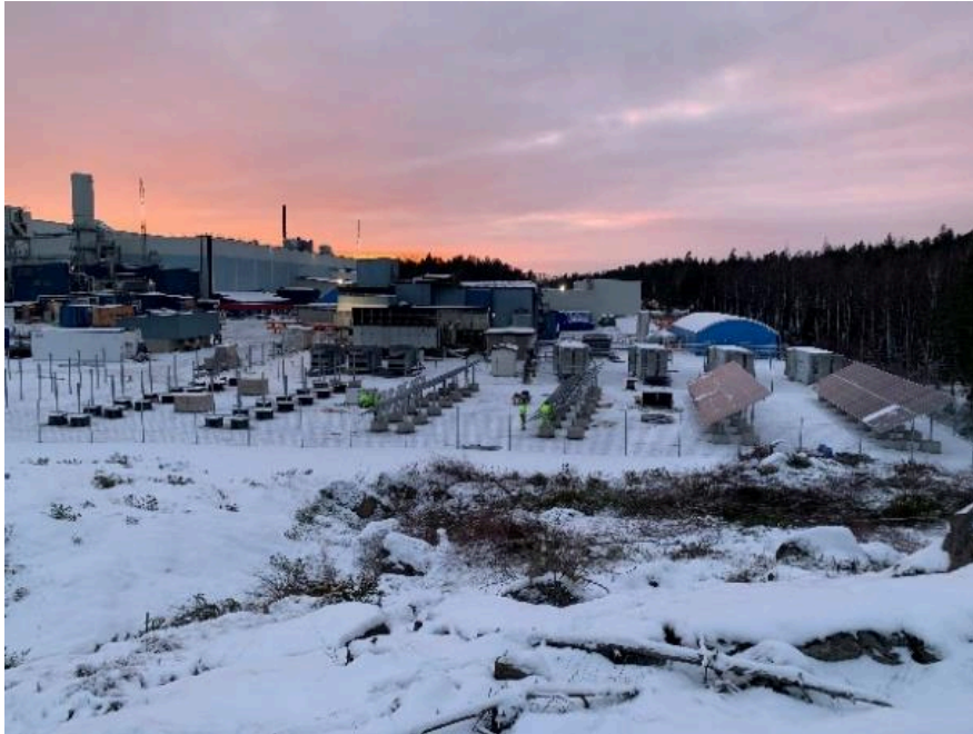
Solar panels installation start winter 2021
